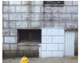
[1] A test patch should always be done before using a chemical cleaner to ensure that it will not damage historic masonry, as in this instance, terra cotta.
