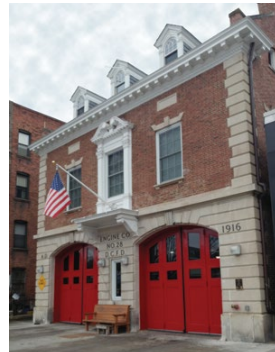
[56 a-b] In order to continue in its historic use, the door openings of this 1916 Colonial Revival-style fire station had to be widened to accommodate the larger size of modern fire trucks. Although this resulted in some change to the arched door surrounds, it is minimal and does not negatively impact the historic character of the building. (a) Above, before; Photo: Fire and Emergency Medical Services Department (FEMS), Washington, D.C.; below, after.
