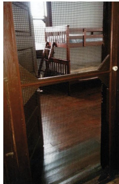
[31] An interior screen door at the entrance to individual apartments is a historic feature traditionally used to help circulate air throughout the building.
