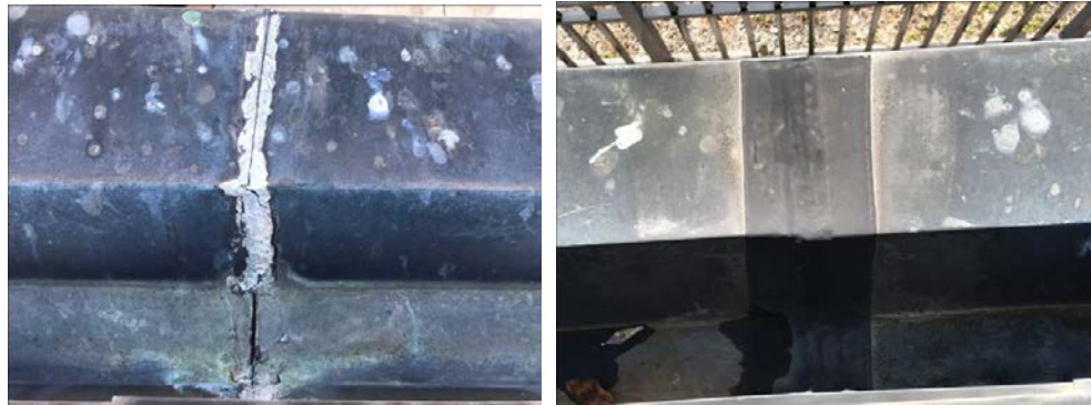
Copper Built-In Gutter Joints
