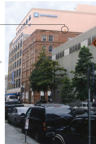
[63] (a) A mockup should be erected to demonstrate the visibility of a proposed rooftop addition and its potential impact on the historic building. Based on review of this mockup (orange marker), it was determined that the rooftop addition would meet the Standards (b). The addition is unobtrusive and blends in with the building behind it.
