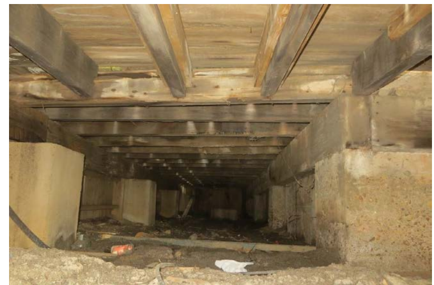
10. Wood Deck Full-Cut Joists with Modern Lumber Partial Reinforcement
