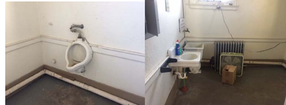
Church Street end of building plumbing fixtures
