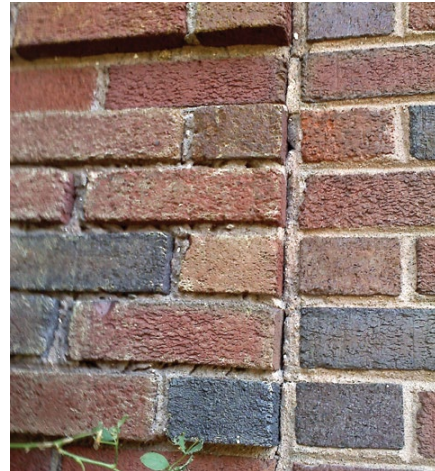
[3] Not Recommended: The white film on the upper corner of this historic brick row house is the result of using a scrub or sturry coating, rather than traditional repointing by hand, which is the recommended method.
