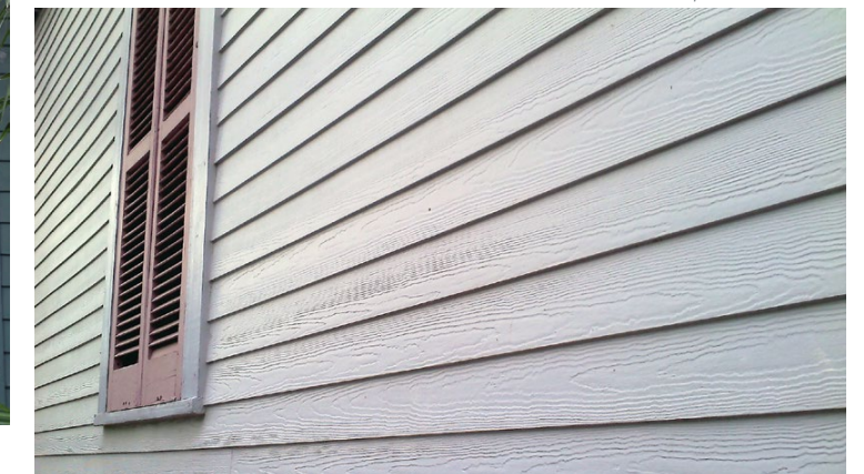
[10] Not Recommended: Cementitious siding with a raised wood-grain texture is not an appropriate material to replace historic wood siding, which has a smooth surface when painted.
