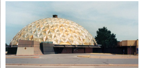
[13] The gold-colored, anodized aluminum geodesic dome of the former Citizen's State Bank in Oklahoma City, OK, built in 1958 and designed by Robert Roloff, makes this a distinctive mid-20th century building.
