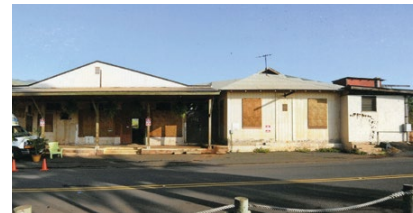
[29] The rehabilitation of the 1910 Māhālaea General Store (a), which served the workers' camp at the Wailuku Sugar Company on the Hawaiian island of Maui, included the reconstruction of the original parapet (b).
