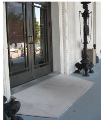
[26] A temporary ramp—unobtrusive and easily removed—facilitates access to the entrance of this museum and does not affect its historic character.
