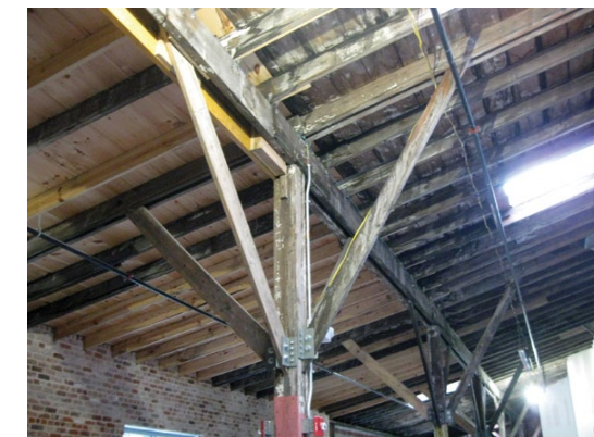
[17] New wood elements have been used selectively to replace rotted wood on the underside of the roof in this historic warehouse.
