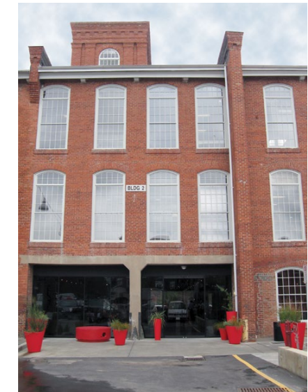
[25] The new infill designs for the garage door openings in this commercial building (a) converted for restaurant use and in this mill building (b) rehabilitated for residential use are compatible with the historic character of the buildings.
