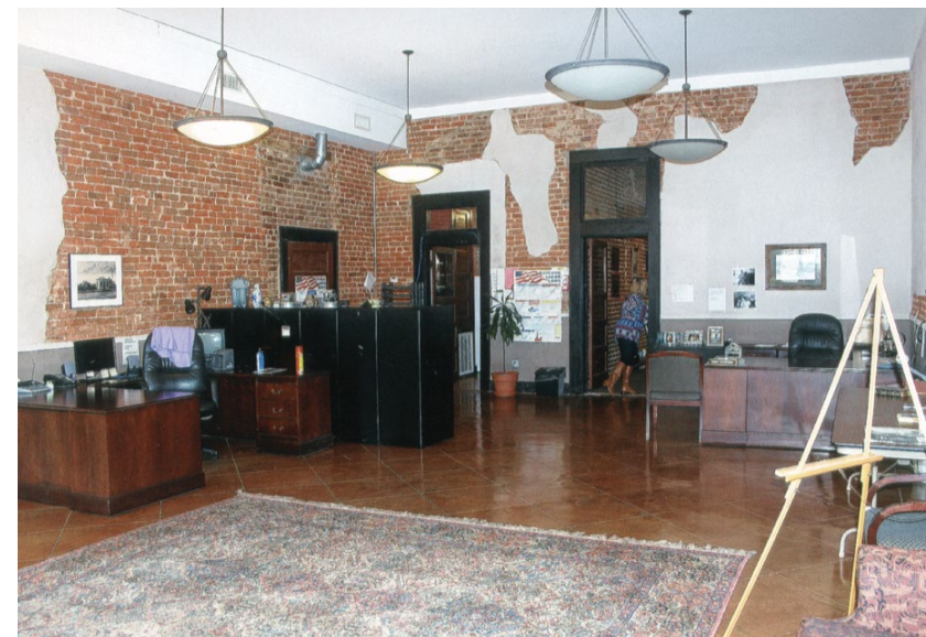
[41] Not Recommended: Leaving fragments of deteriorated or "sculpted" plaster is not a compatible treatment for either finished or unfinished interior spaces.
