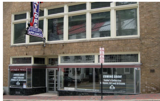
[15] Regular maintenance has helped to preserve this historic storefront, which retains all of its character-defining features, including the granite bulkhead, multi-paned transom glazing, and recessed entrance.
