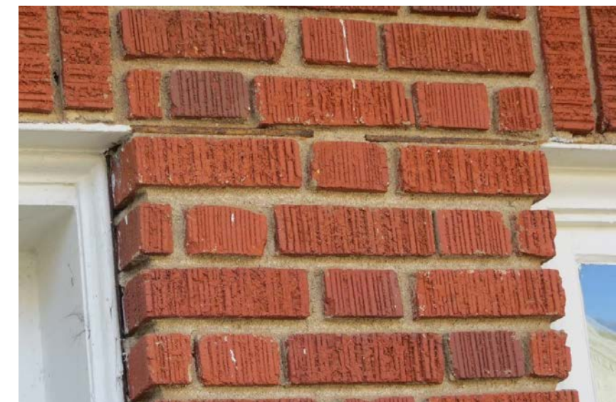
6. Exposed Rusty Steel Lintels with No Mortar Cover
