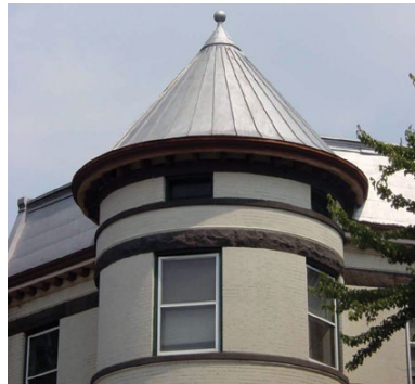
[6] A standing-seam sheet metal roof, like the one on the turret of this late 19 th century row house, must be kept painted to ensure its preservation.
