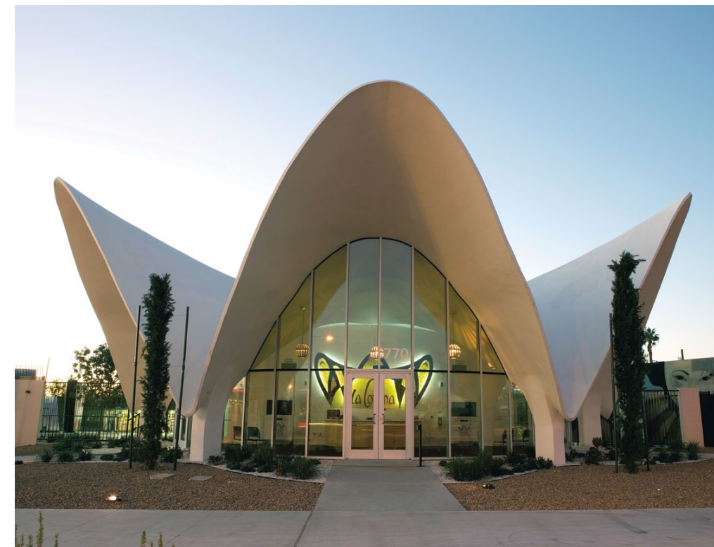
[2] Mid-century modern building technology made possible the form of this parabolic-shaped structure and its thin concrete shell construction. Built in 1961 as the lobby of the La Concha Motel in Las Vegas, it was designed by Paul Revere Williams, one of the first prominent African-American architects. It was moved to a new location and rehabilitated to serve as the Neon Museum, and is often cited as an example of Google architecture. Credit: Photographed with permission at The Neon Museum, Las Vegas, Nevada.
