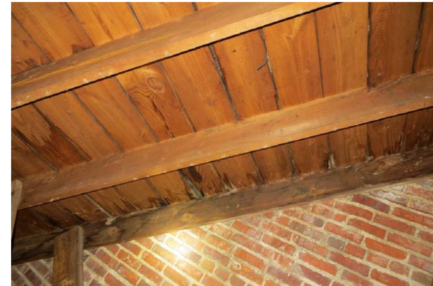
1. Roof Trusses East of Firewall Above Ceiling
