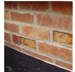
[2] Not Recommended: The use of inappropriate Portland cement mortar to repoint these soft 19th-century bricks has caused some of them to spall. Photo: Courtesy Nebraska State Historic Preservation Office.
