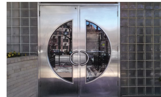
[1] The stainless steel doors at the entrance to this Art Deco apartment building are important in defining its historic character and should be retained in place.
