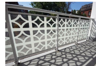
[59] (a-b) The decorative concrete balcony railings on this 1960s building did not meet life-safety code requirements. They were replaced with new glass railings with a fritted glass pattern matching the original design—a creative solution that satisfies codes, while preserving the historic appearance of the building when viewed from the street (c-d). Photos: (a, b, d) ERA Architects, Inc.; (c) Nathan Cyprys, photographer.
