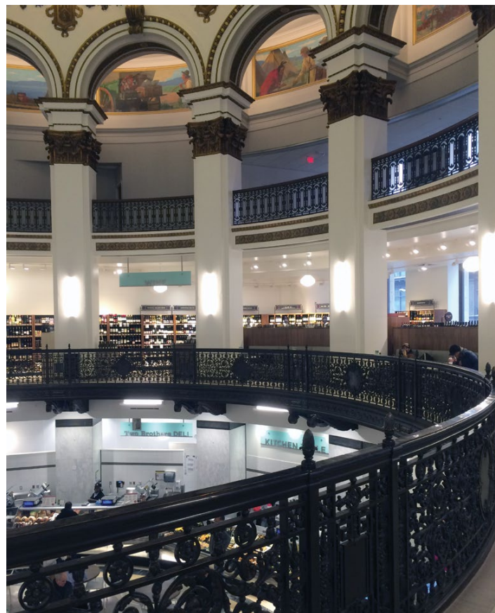
[36] The elaborate features and finishes of this historic banking hall in the Union Trust Company Building, in Cleveland, OH, were retained and repaired as part of its conversion into a food market.
