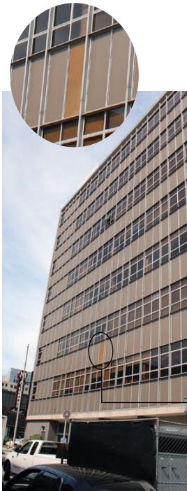
[16] Plywood provides temporary protection for an opening where a damaged spandrel panel was removed until a matching replacement panel can be installed.
