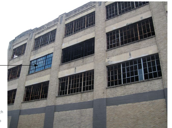
[18] The historic metal storm windows in this 1920s office building were retained and repaired during the rehabilitation project.
