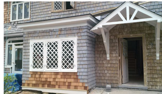
[5] Rotted wood shingles have been replaced in kind with matching wood shingles.
