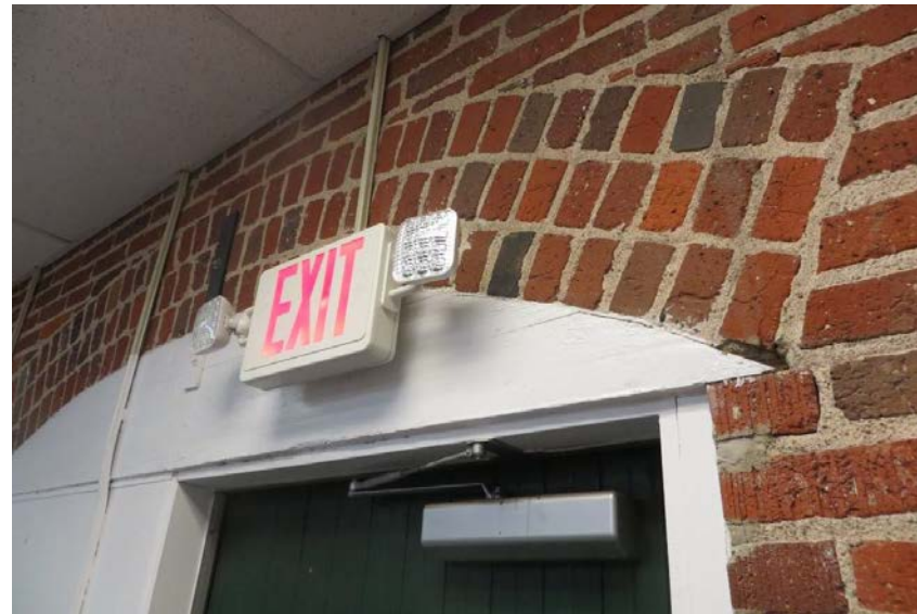
7. Typical Interior 8" Brick Arch at Door and Window Openings
