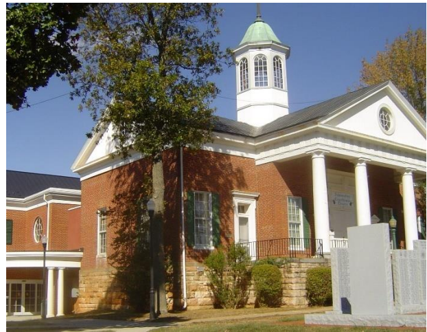
Appomattox County Courthouse Image Source: Wikipedia Commons
