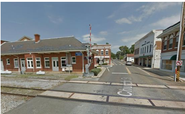
Church Street Facing North – Existing Conditions Image Source: Google Maps
