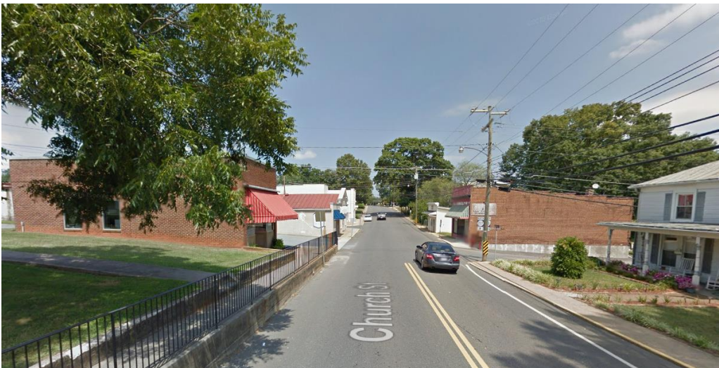
Church Street – Existing Conditions Image Source: Google Maps
