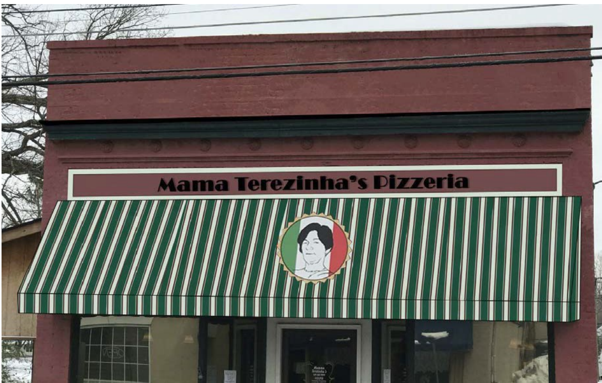
Example of a Façade Improvement from a Preliminary Work Write-Up for Mama Terezinha's Pizzeria
