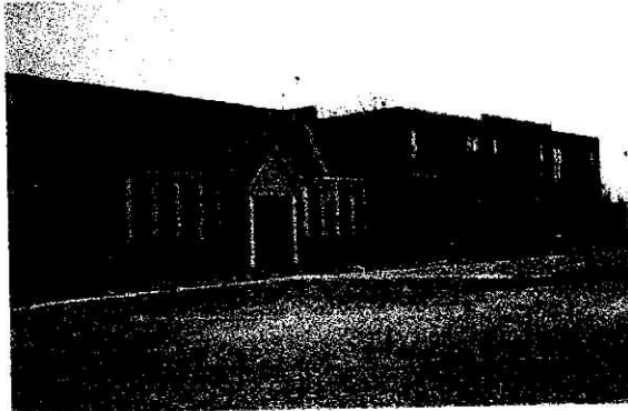
Appomattox Elementary School The wing on the left is the original Carver Price School
