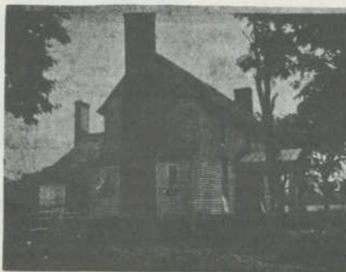
BEFORE RESTORATION - Photo taken in June of 1972. Although roof and timbers were sound the house was in a bad state of repair.
